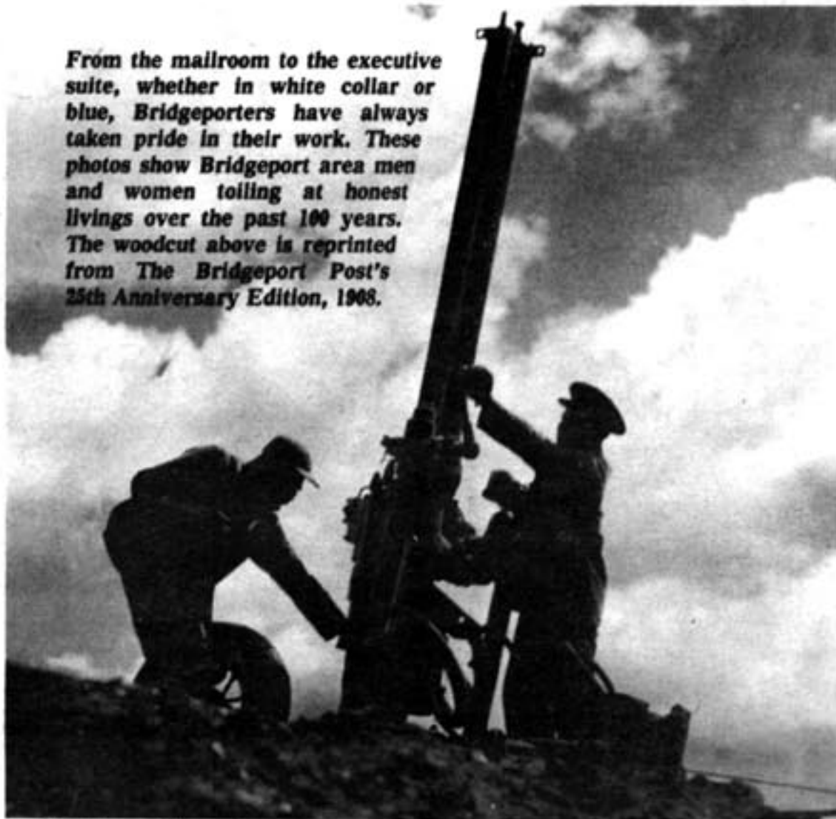
Pile drivers strike an heroic stance during construction of the Connecticut Turnpike in Bridgeport in 1956. Post photo by Al Mathewson.
