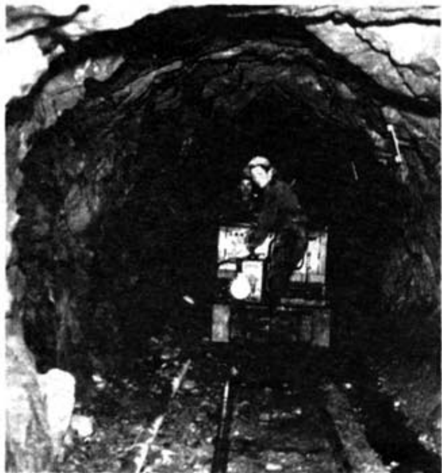
Bridgeport Hydraulic Company workers tunneled 7,100 feet below the solid rock of Popp's Mountain on the Easton-Weston town line to connect the Saugatuck and Aspetuck reservoirs in the 1930s and 1940s. Courtesy of Bridgeport Hydraulic Company.
