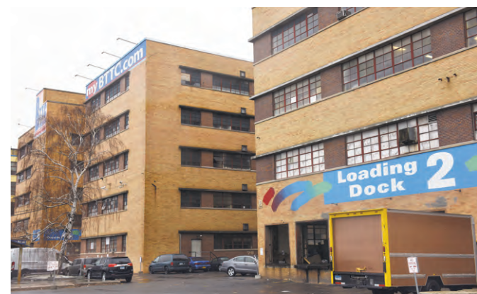
Modify Furniture in the BTTC building in Bridgeport.
